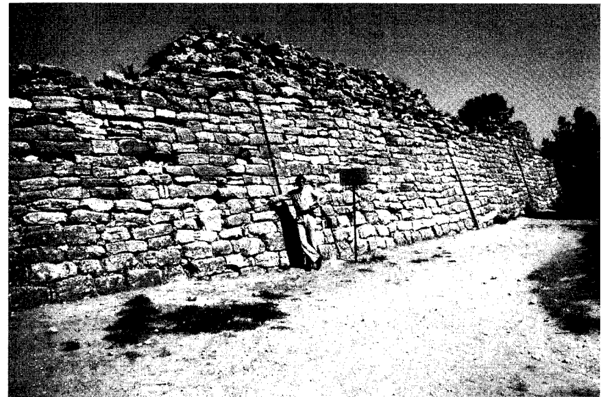
Figure 10. The author before the walls of Troy, from level VI, c. 1250 BC. The finely built walls incline slightly inward and are reinforced by vertical batters at regular intervals. Photo © the author
